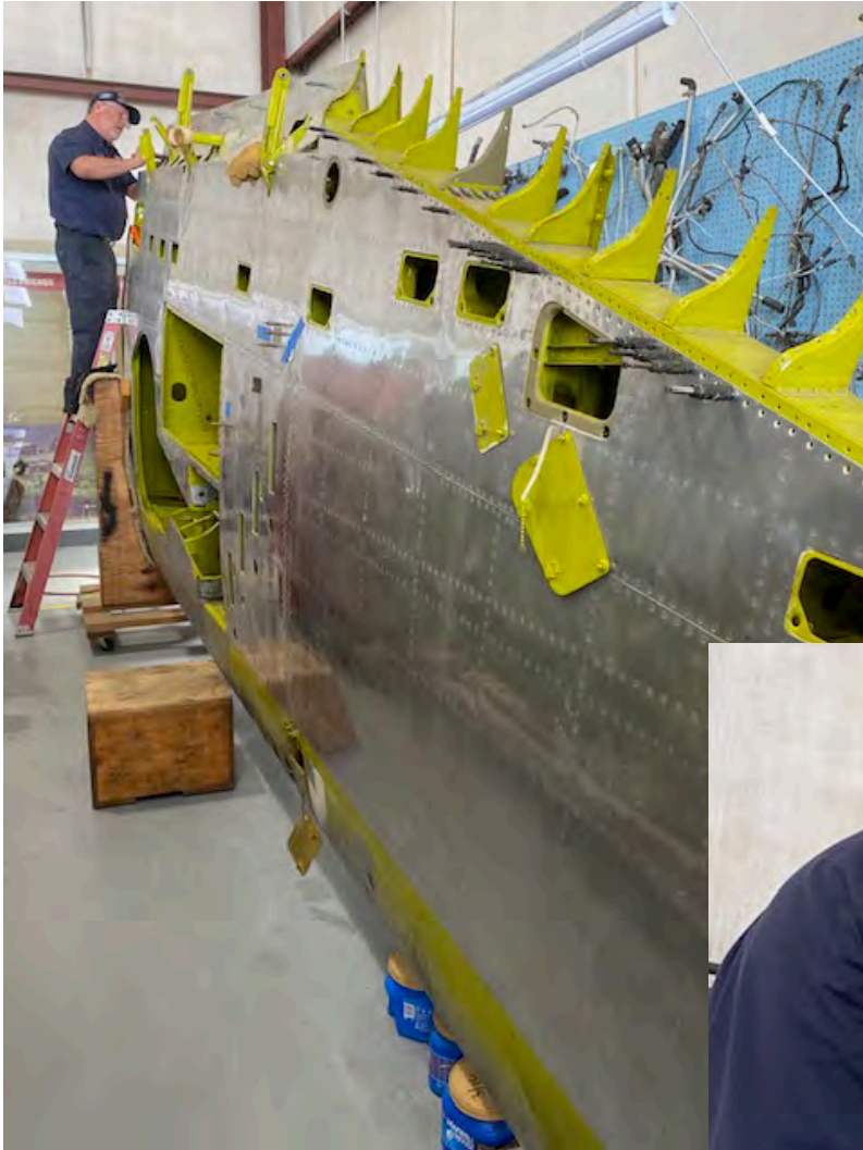
Col Steve Barnshaw does sheet metal repair on one of the wings of the P-47.
