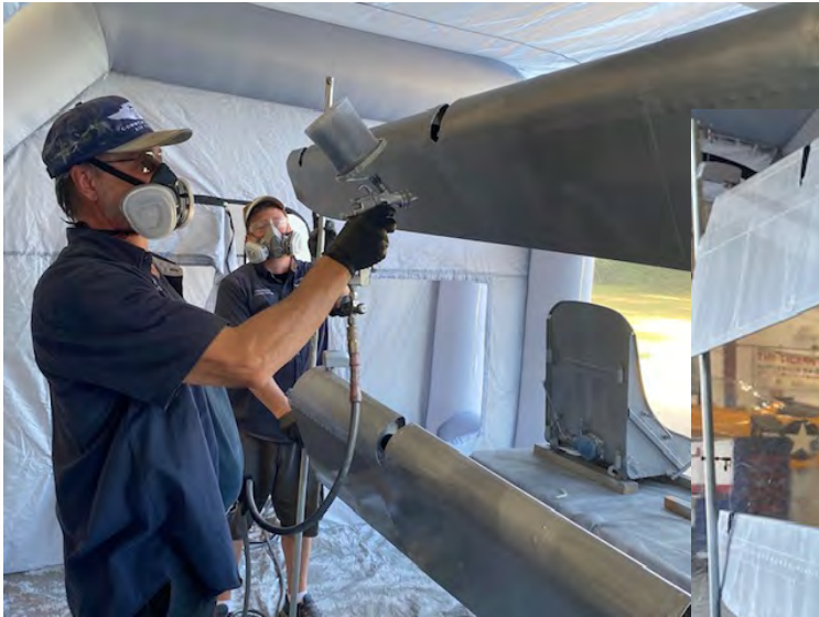
Above and Right: Cols Handler & Buzzeo painting the PT-19 ailerons.
